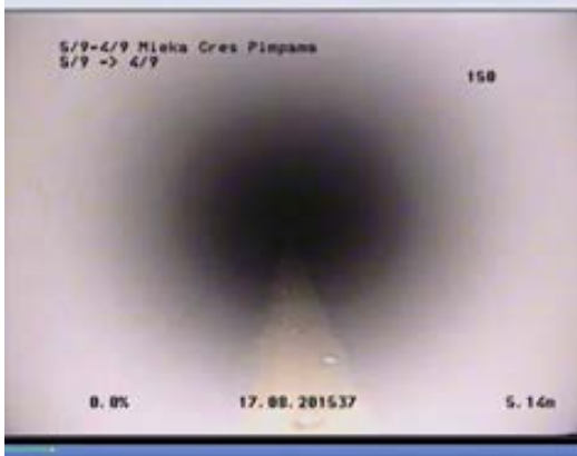
FIG A8.3: Example of a minor deposits at the invert – acceptable
