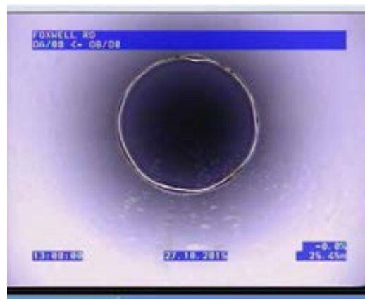
FIG A5.4: Example of a defective house junction – not acceptable FIG A5.5: Example of a defective joint – not acceptable
