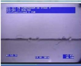
FIG A5.2: Example of defects at a joint – not acceptable
