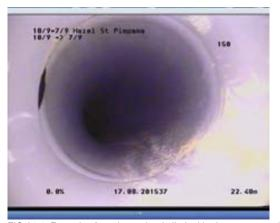
FIG A6.1: Example of an obstruction (rolled rubber) – not acceptable
