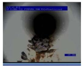
FIG A8.5: Example of a major deposits at the invert – not acceptable FIG A8.6: Example of a deposits in a junction – not acceptable
