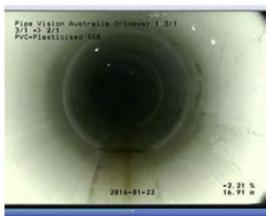
FIG A7.1: Example of minor ponding within a pipe – acceptable
