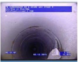
FIG A6.4: Example of an obstruction within a pipe – not acceptable
