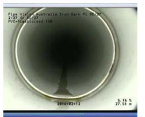
FIG A5.8: Example of excessive width at a joint - not acceptable
