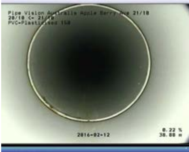
FIG A5.7: Example of a well constructed joint – acceptable
