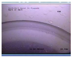
FIG A5.9: Example of excessive width at a joint - not acceptable
