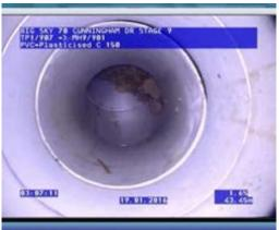
FIG A8.7: Example of a deposits in a junction - not acceptable.
