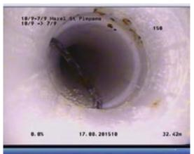
FIG A6.2: Example of an obstruction (rolled rubber) – not acceptable
