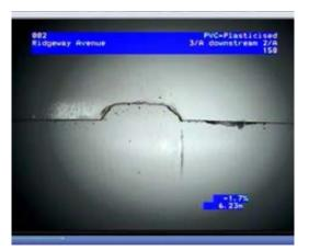
FIG A5.1: Example of a defect at a joint – not acceptable
