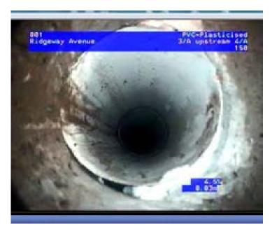
FIG A5.6: Example of a defect at the manhole/pipe interface joint – not acceptable
