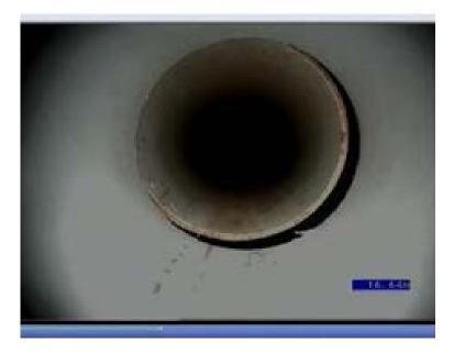
FIG A4.1: Example of collapse at a joint – not acceptable
