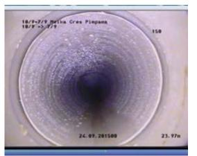
FIG A5.10: Example of excessive gap at a coupling - not acceptable
