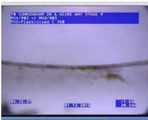
FIG A1.3: Example of poor quality footage of a joint - not acceptable
