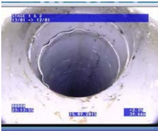
FIG A5.4: Example of a defective house junction – not acceptable FIG A5.5: Example of a defective joint – not acceptable
