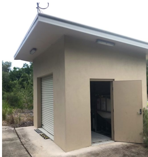
Figure 1: Example of typical standards MHL Dosing building
