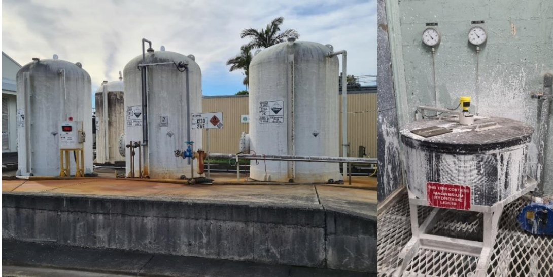
Figure 16. Make pressure washing the preferred option to clean equipment, rather than chemical treatments. MHL tanks (shown right) are messy, so provide splash shields.
