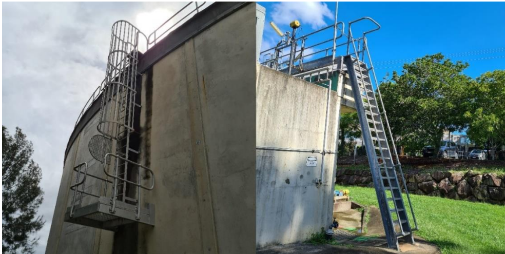
Figure 7. Ladders provide access to roofs, equipment, and instruments.
