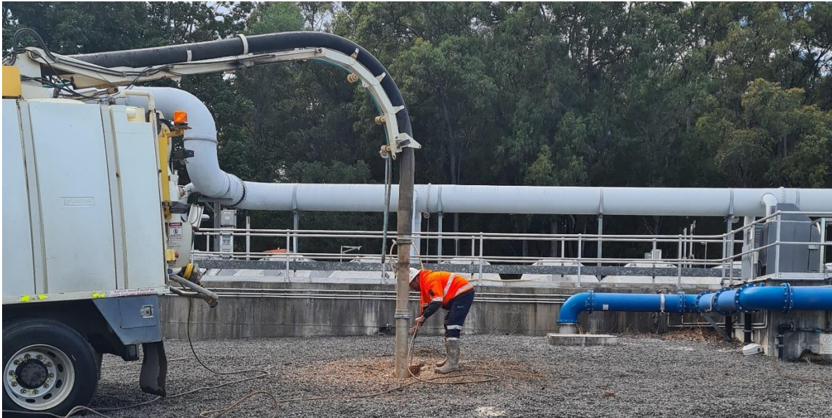
Figure 22. Pipes and conduits under gravel can be investigated when issues arise, without impacting site access.
