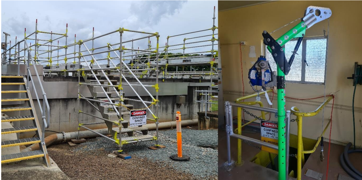
Figure 15. Ensure scaffolds, signs, rescue kits and davits can be set up at entrances.
