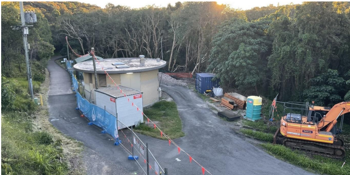
Figure 18. Divert pedestrians to give enough working space for construction activities.
