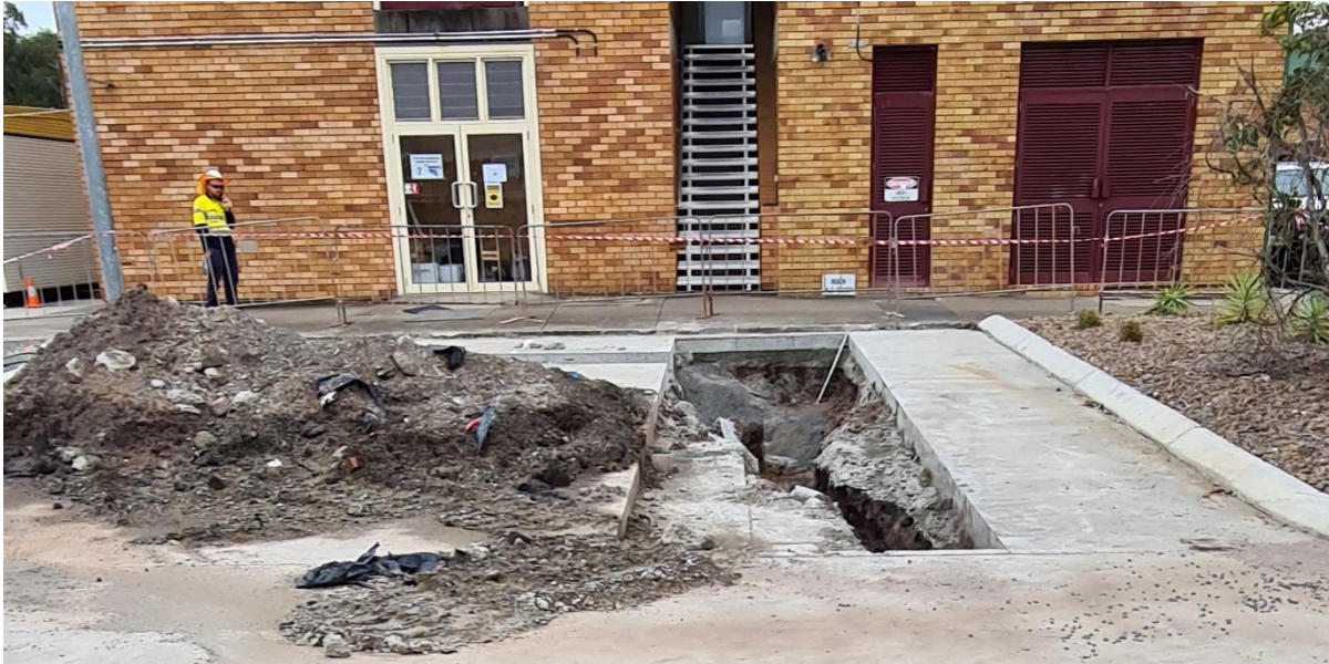
Figure 23. Digging trenches to investigate infrastructure under hard cement laydowns.
