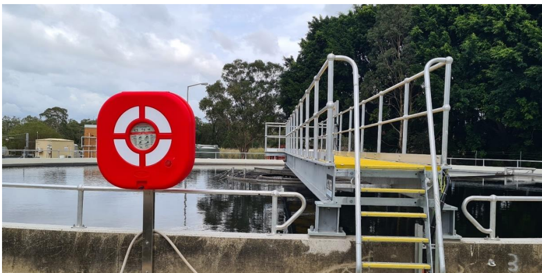
Figure 9. Handrails around clarifiers reduce the risk of working near water.
