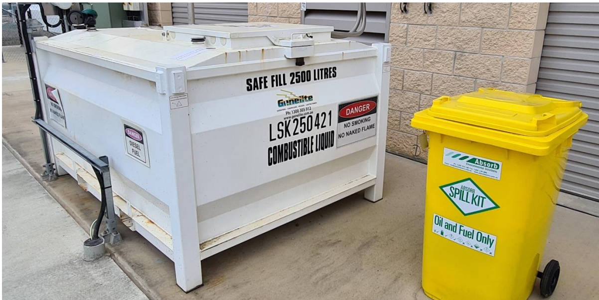
Figure 20. Combustible diesel fuel stored in an open area away from process plant.
