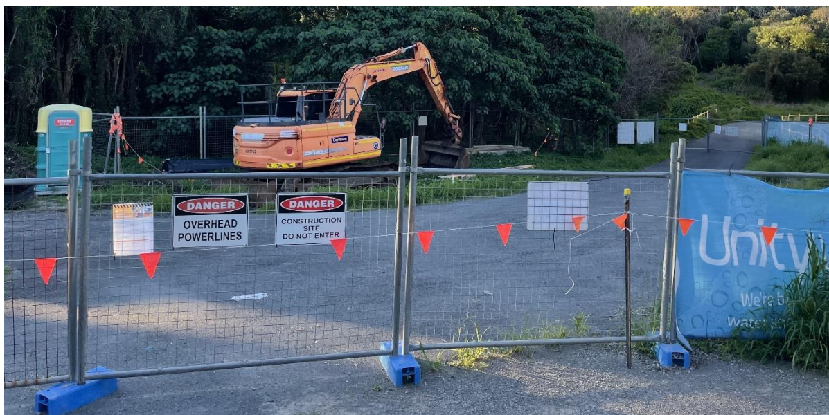
Figure 19. Constructing pedestrian bypasses can limit public safety impacts.
