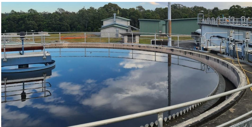
Figure 8. Only limited interactions are performed on the path beside this clarifier.
